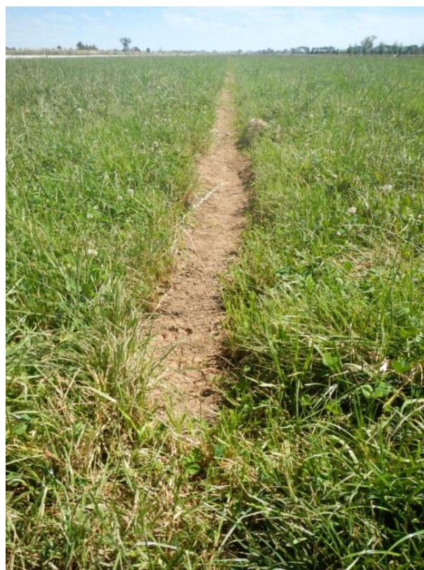
Figure 3: Shallow surface drain installed on a pasture bay
