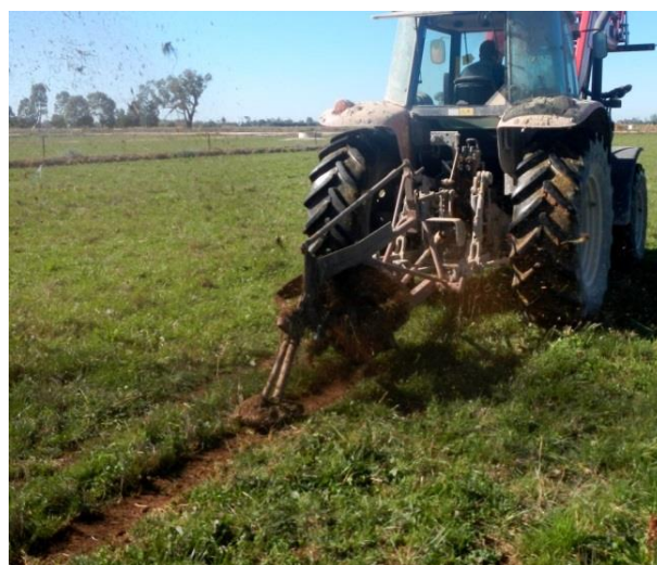
Figure 4: Surface drain installation
